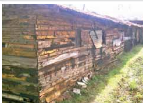
Police accommodation at Kerugoya Police station
